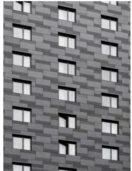
Designers collaborated with TAKTL to fabricate dual-textured molds, cast in one standard color, and ColorSealed to accentuate the textural variation and minimize color differences panel to panel.
