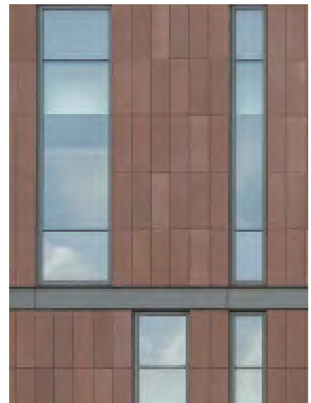
Natural color variation stems from variances in natural raw materials. Small differences in sand and cement coloration still can result in panel to panel or lot to lot color variation.
