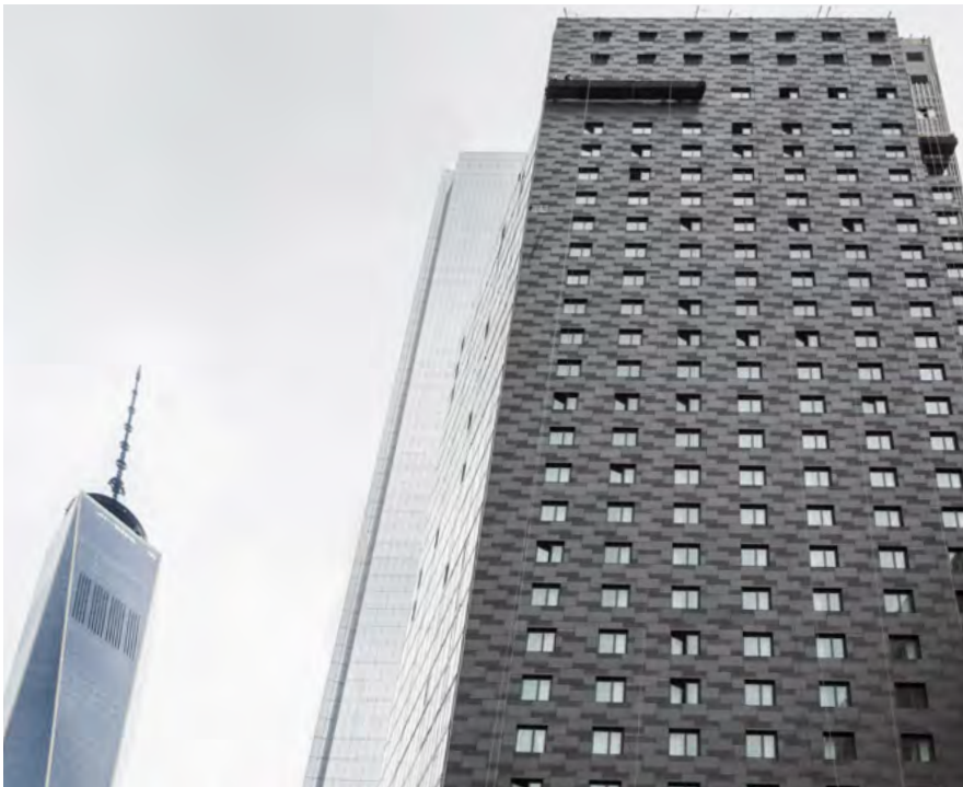
Designers collaborated with TAKTL to fabricate dual-textured molds, cast in one standard color, and ColorSealed to accentuate the textural variation and minimize color differences panel to panel.
