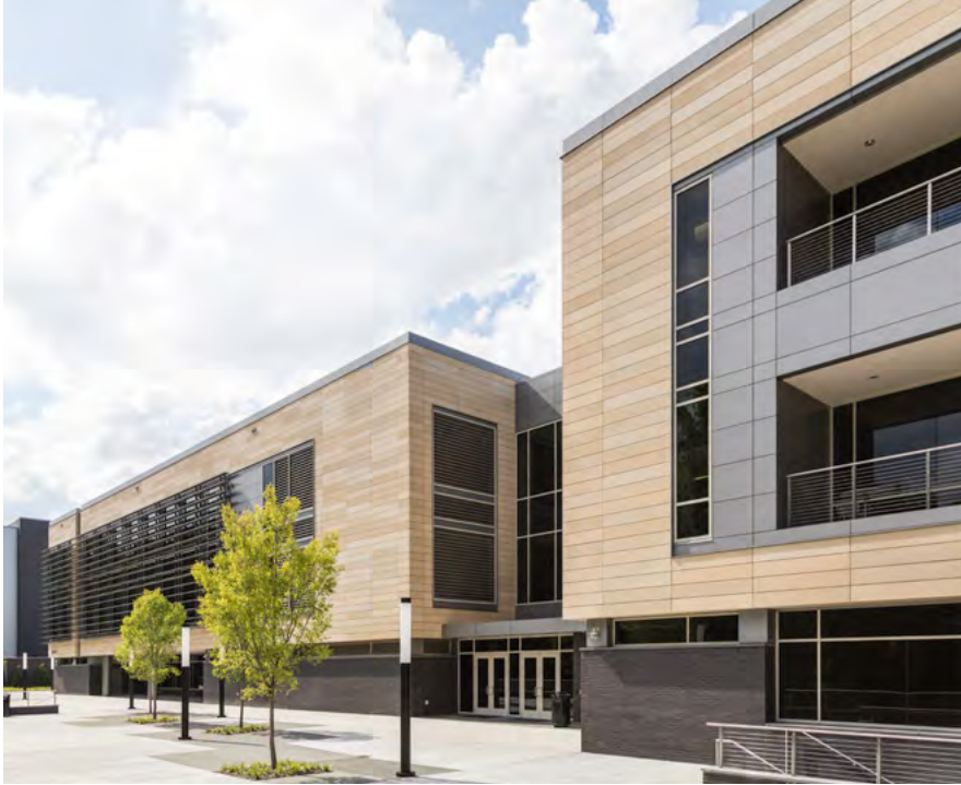
Designers have successfully incorporated two standard textures, cast in one custom color, to create random variation across the elevations.
