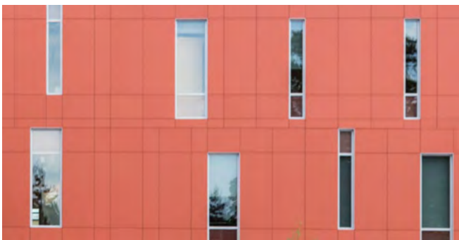
Saturated colors can display extreme variation in different lighting conditions. ColorSeal should be specified if color variation is not desired.
