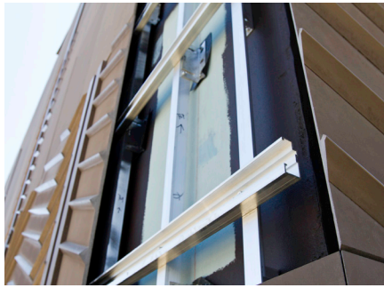
Rainscreen | Undercut Anchors
